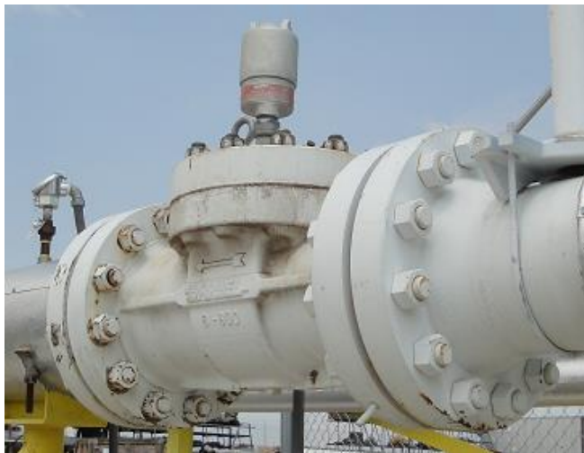
Figure 6 – 8" Turbine Meter
